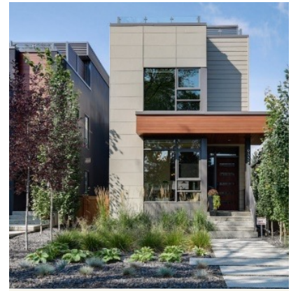
This infill house has a generous front setback which provides space for landscaping and a walkway.
