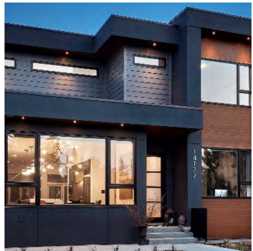
These infill houses include clerestory windows which enhance interior daylighting without creating overlook into adjacent properties.
