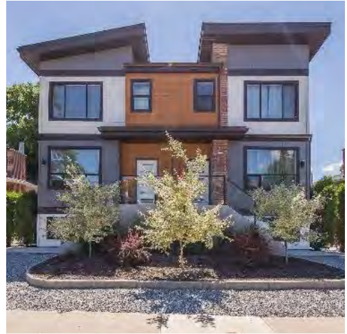
Example of a semi-submerged basement.
