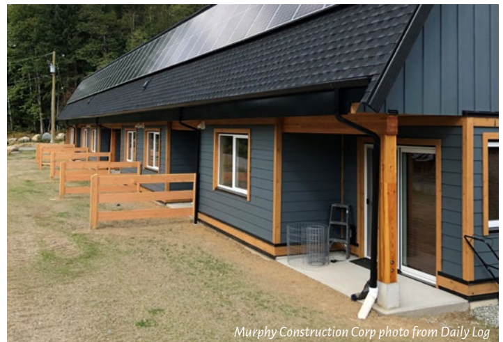
Murphy Construction Corp photo from Daily Log
